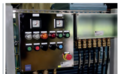
On-Off Operation by Local Control Panel
