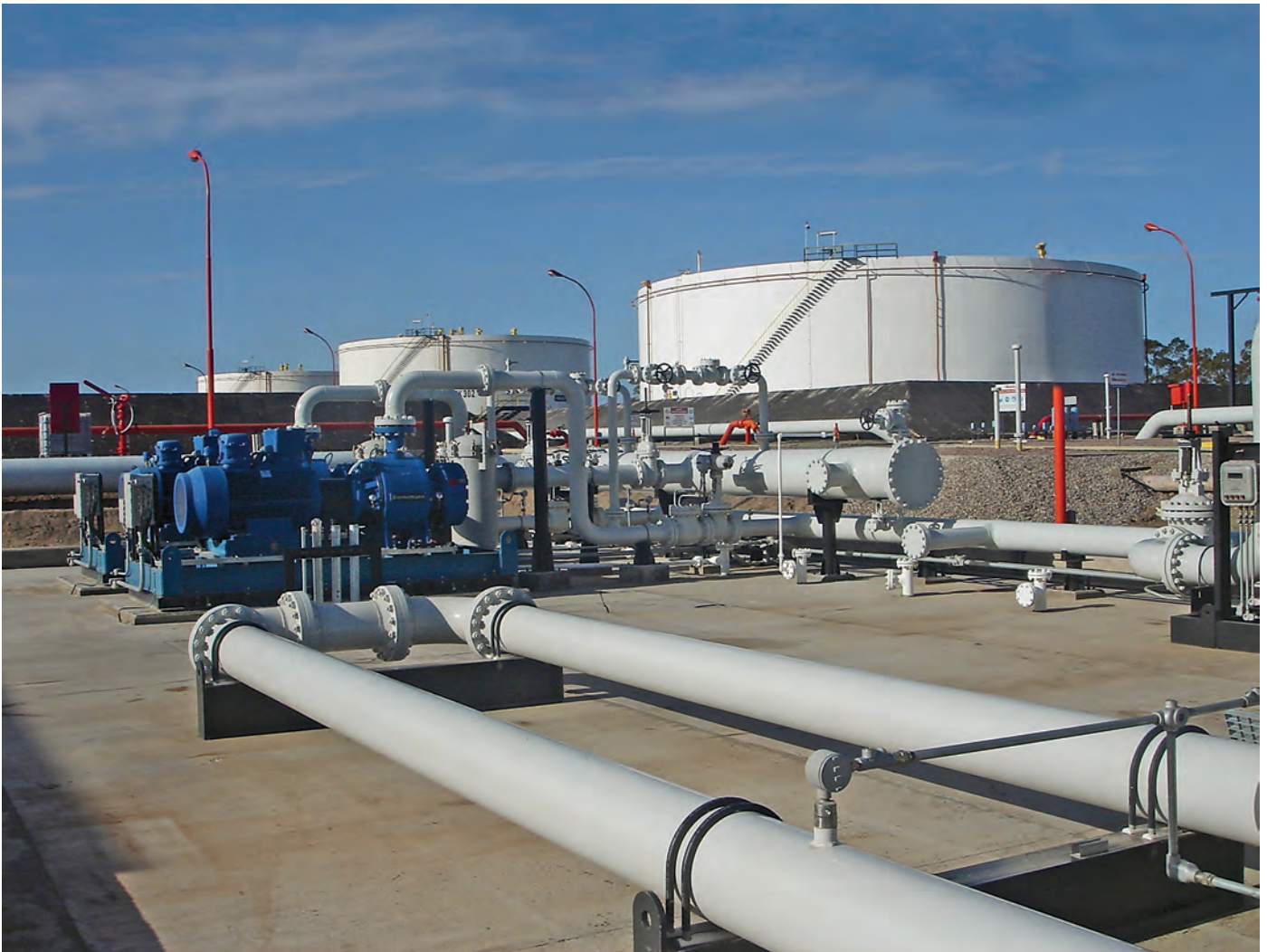
Onshore Terminal in Argentina
